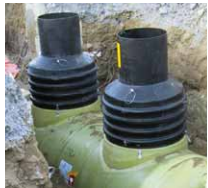
EuroHUK maintenance shafts installed.
