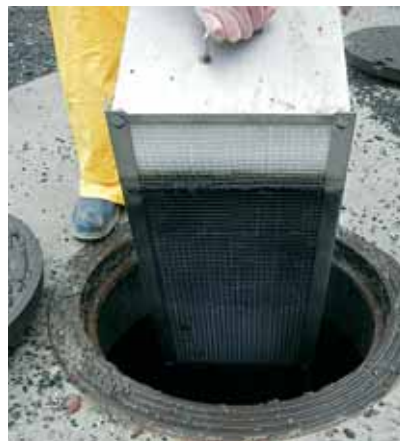
Coalescing unit can be removed for maintenance.
