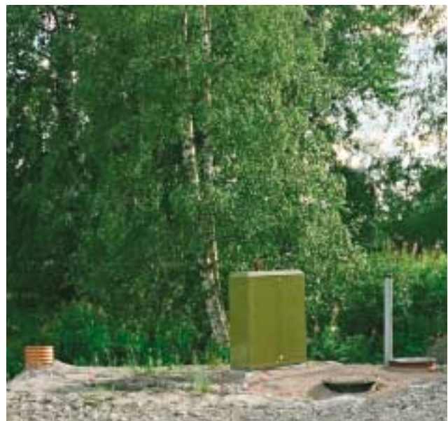
Labko BioKem 30 batch reactor installed.
